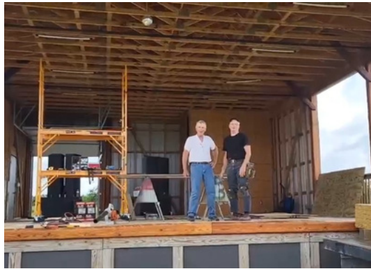
Completing the stage floor with another layer of plywood
